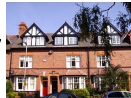
Part of the terrace at 43-55 Springfield Road
